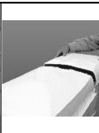
Place the cover on the flange
