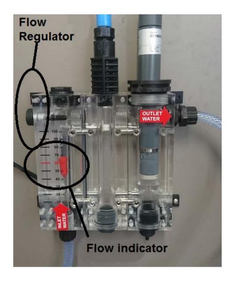
3) Switch on the electrolysis / dosing System. The CL reading will increase slowly, and will be stable after some minutes.
