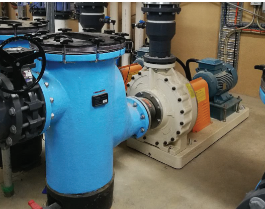
Basket Strainer works with SWP series FRP pump
